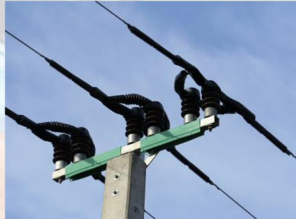
Adequate insulation on a medium voltage poletop (Photo: Zoltán Orbán)
