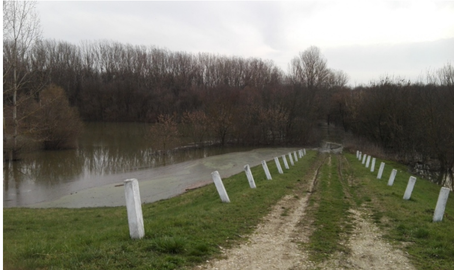
The project site in February 2016 (Photo: Béla Tokody)
